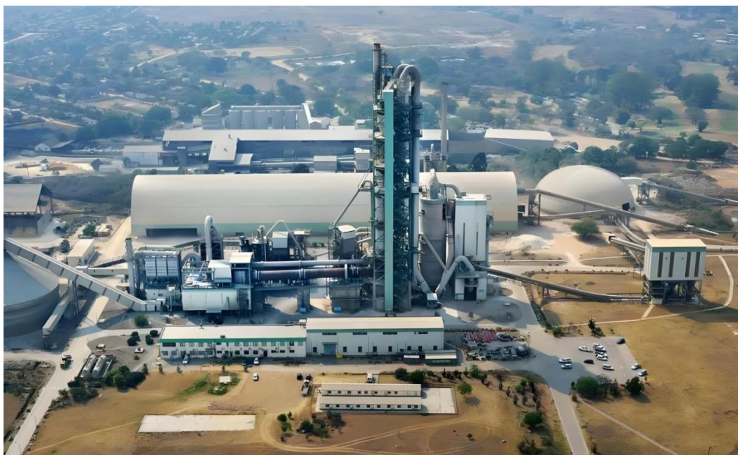
Figure 2: Panoramic View of Huaxin Building Materials Overseas Cement Factory
